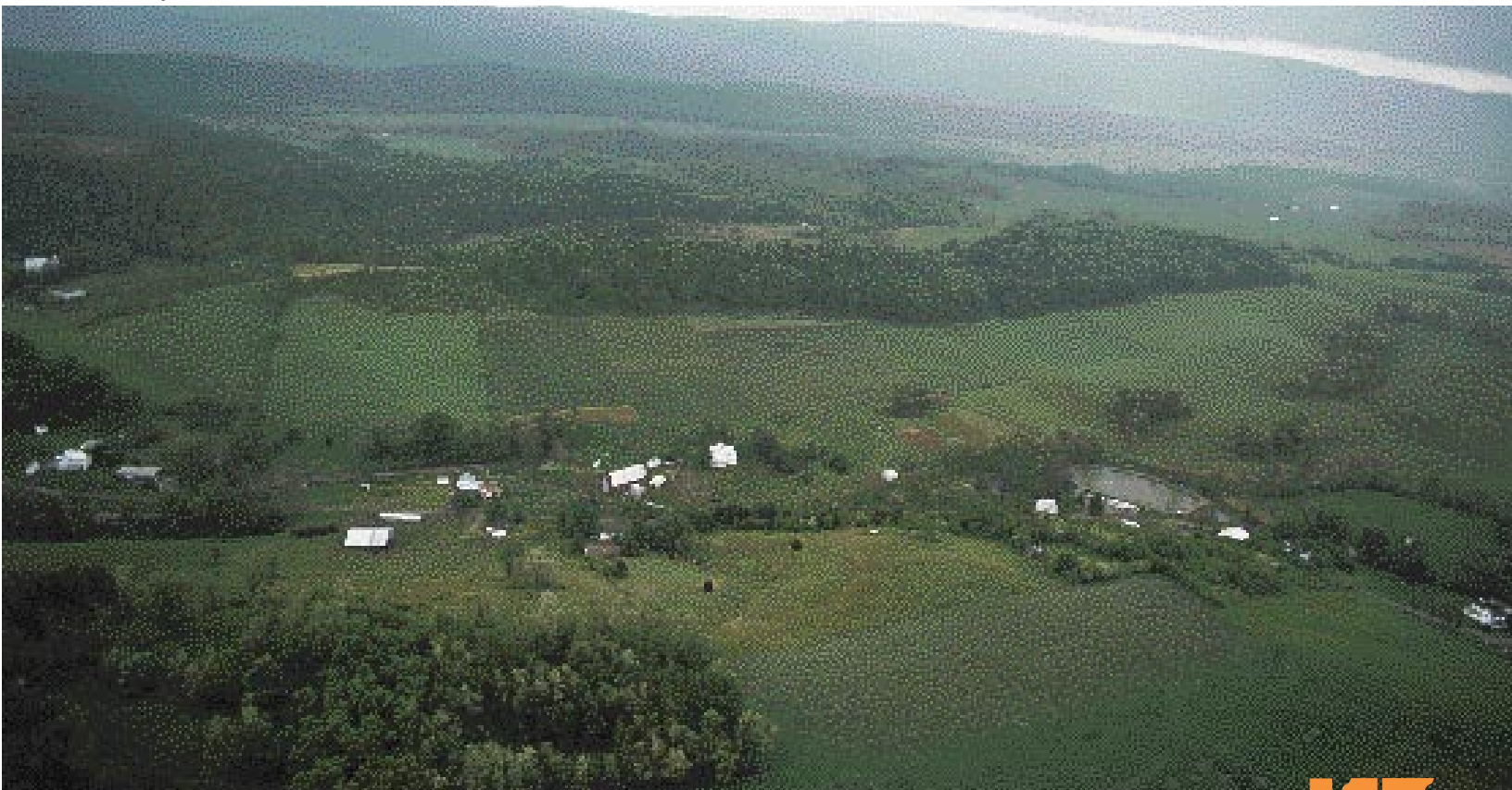
lack of corridors
