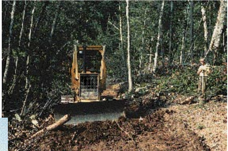
building water bar
